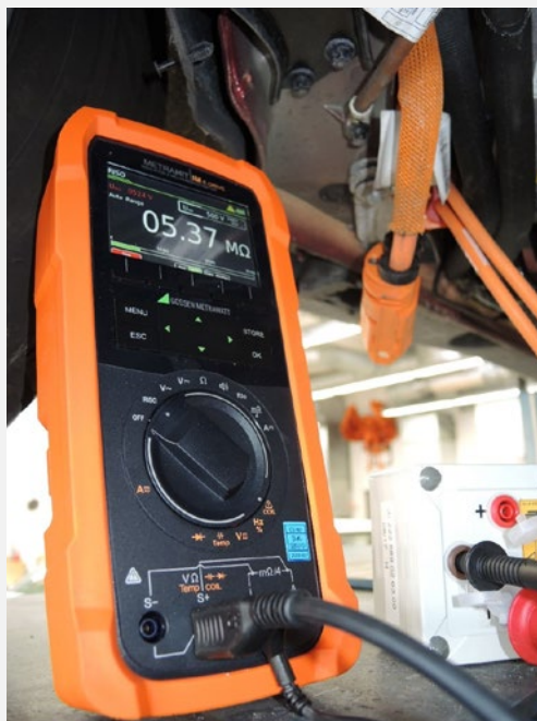
Figure 12: Testing Insulation Resistance with a 500 V Test Voltage Between Inverter and Ground with a Measuring Adapter on the Rosenberger Plug using the Mercedes GLC 350 e as an Example
