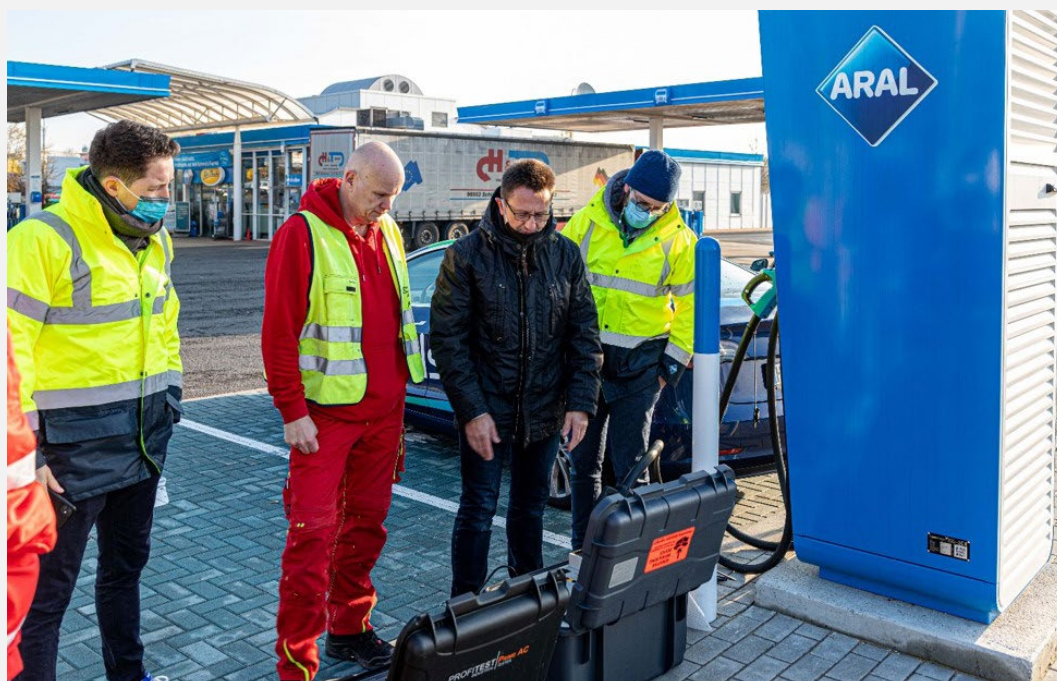
Figure 9: Charging Point Test with PROFITEST H+E XTRA and PROFITEST PRIME
